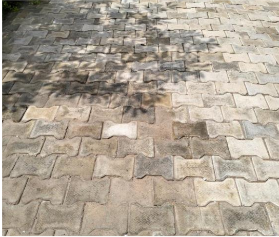
Paving stone installed in campus
